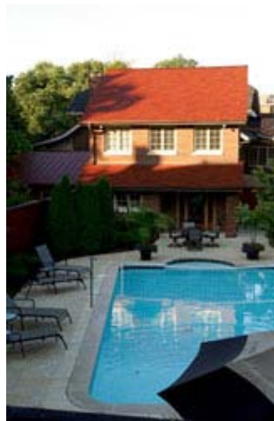
The patio side of this two-story Highlands garage serves as a poolhouse, while the second floor is a woodworking studio.
